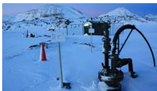
CO 2 injection bore at Hellisheidi.
